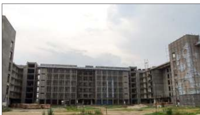
Shri Vishwakarma Skill University – Construction Site
