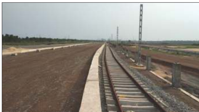
Construction Site- MMLP Paradip (Odisha)
