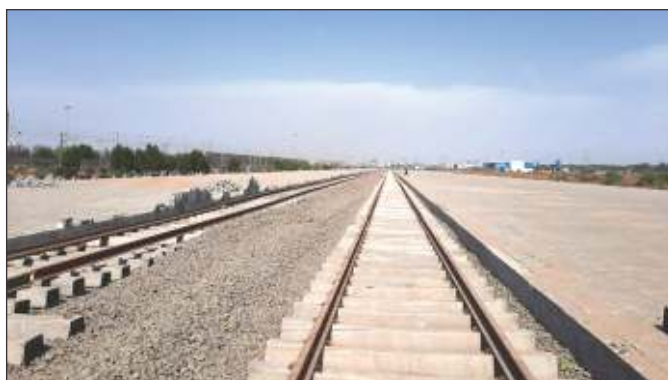
Construction Site- MMLP Dahej, Gujarat
