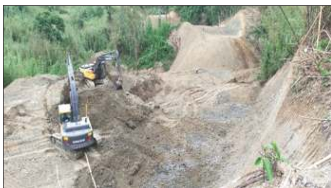
Excavation Work in Progress at Km 103.400 to 103+500
