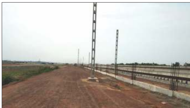
Construction Site- MMLP Paradip (Odisha)
