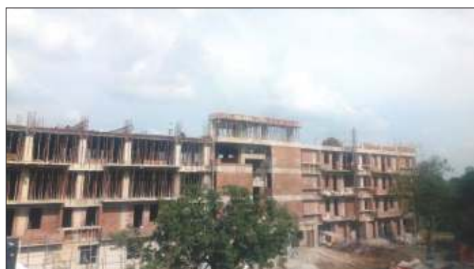
Construction Site – Jogbani, Bihar
