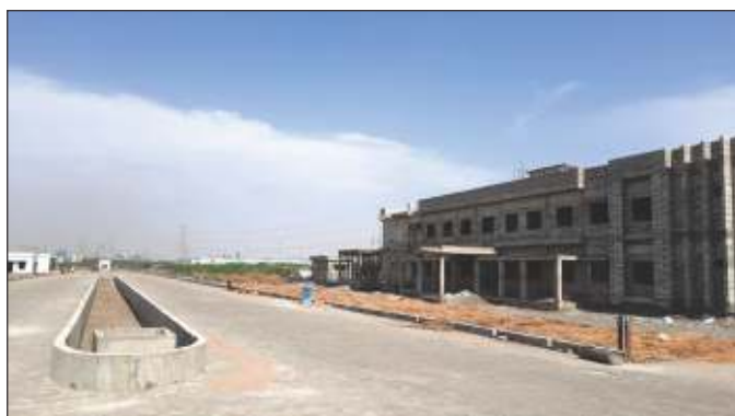
Construction Site- MMLP Dahej, Gujarat
