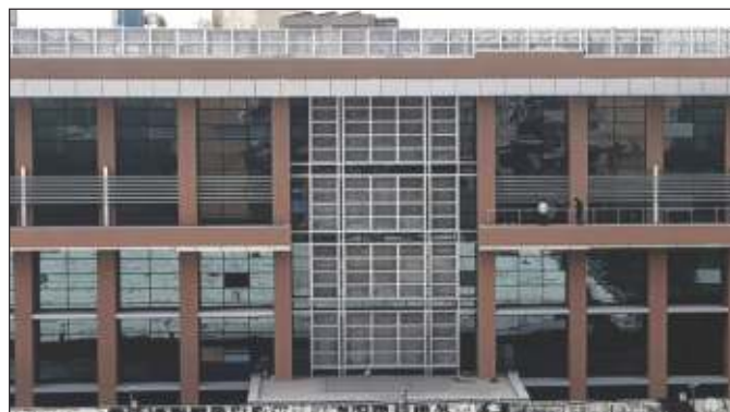
DST – Construction Site
