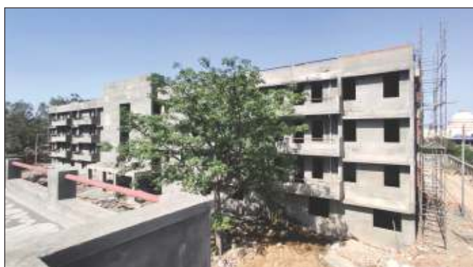
Construction site – Attari, Punjab
